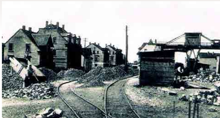
Loading station with stonemason's huts, Beucha around 1900
