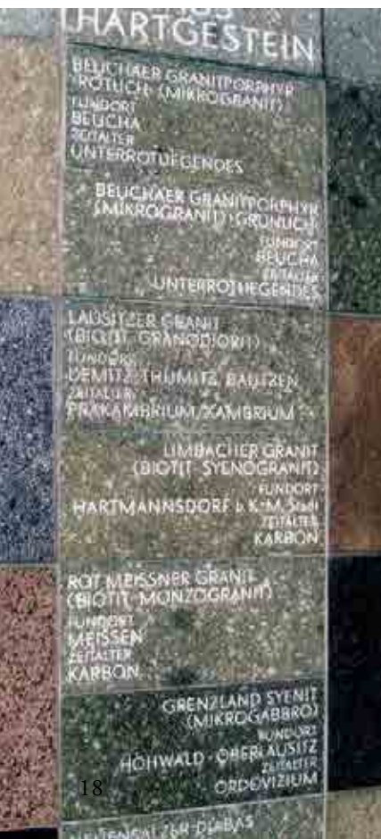
Concrete column at the Kirchbruch Beucha, lined with dimension stones cut from Saxon rocks
